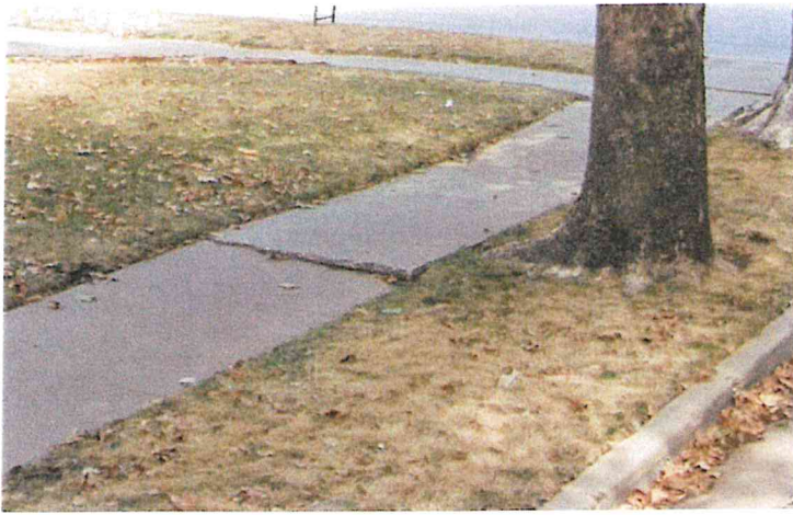
Trip hazard moving east along east-west sidewalk section. Tree root likely cause of pushing up the sidewalk.
