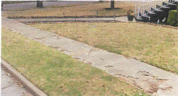
Sidewalk is approximately 1"-2" in locations along the west curb line of Lee Ave. that can be pulled up and inspected. Various pieces missing within existing panels.
