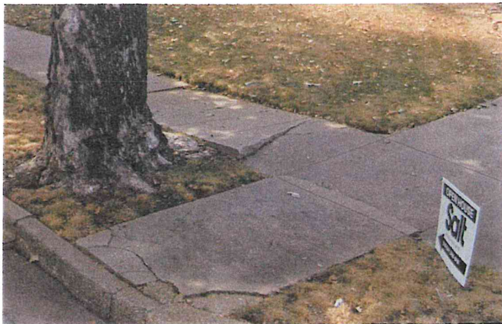
Trip hazard at panel just west of intersection of east-west/north-south sidewalks. Tree root likely cause of pushing sidewalk up.
