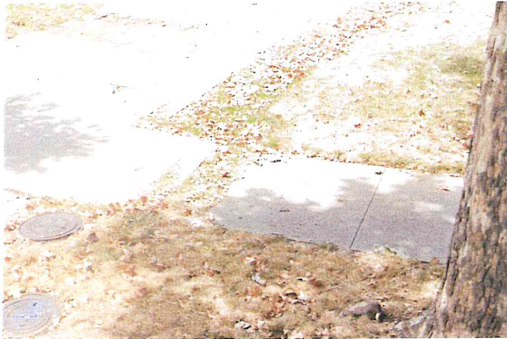
Missing section of sidewalk likely due to utility work to run new service line to neighbor's house north on Lee Ave.
