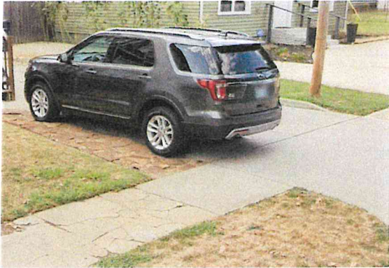
Existing panel adjacent to new driveway and sidewalk concrete is cracked.
