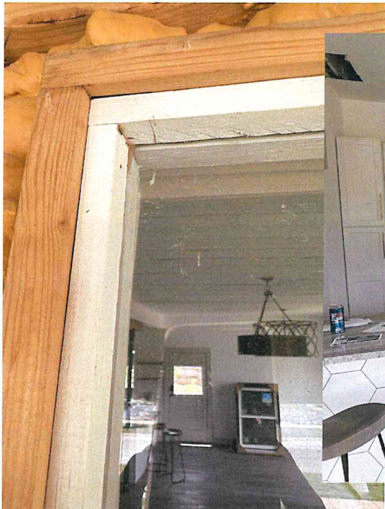
SITE BUILT WINDOW FRAME. \frac{1}{8} " GLASS SANDWICHED BETWEEN 2-1x1 FRAMES, FASTENED TO OUTSIDE 2x4 FRAME
