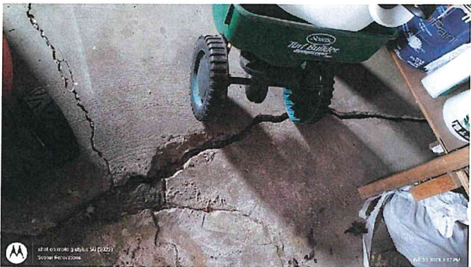
Garage concrete has extensive damage
