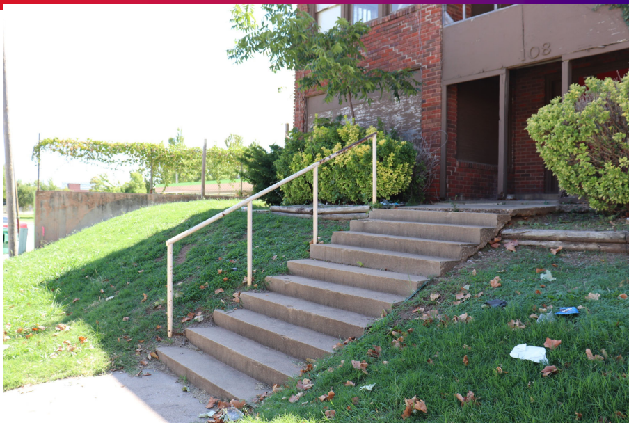
Steps Leading to Front Entry at North Elevation; Note Failing Slope or Terrace
