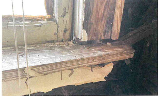
A typical window frame and sill. Windows frames are very rotted, and many have been nailed or painted shut.
