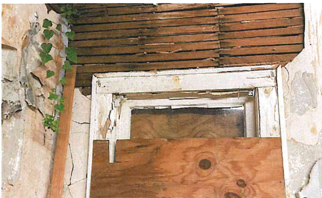
Board removed to exposed boarded up window below. Similar condition to other windows. Assumed first floor windows all boarded up for security.
