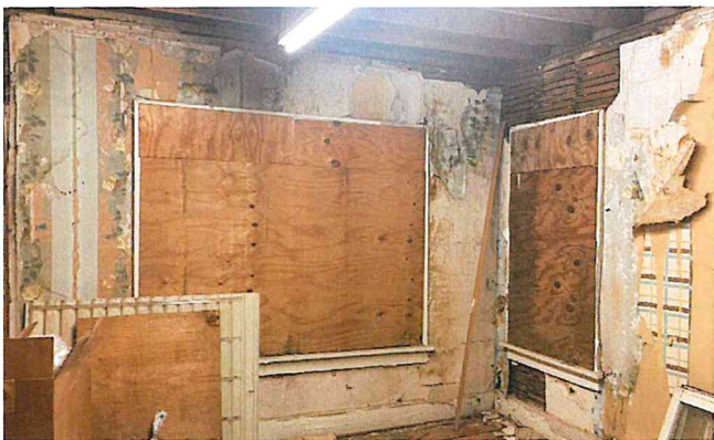
Many windows have been destroyed and boarded up. Basically every first floor window opening is in this condition.
