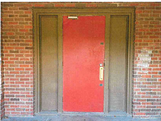
Entry door condition. Door and Side-Lites to be replaced.
