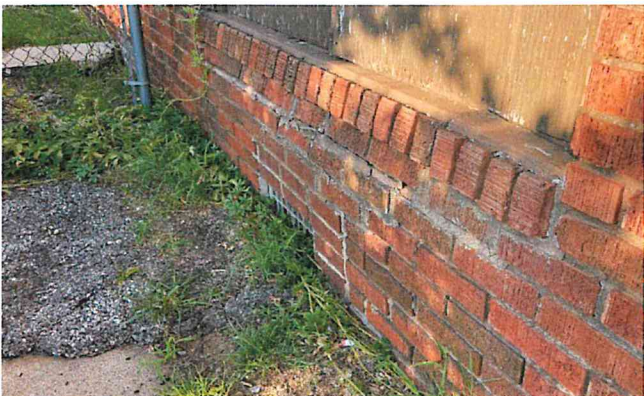
Some brick needs to be repaired. No new brick to be used.
