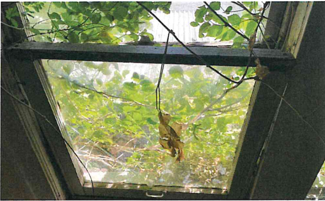
Some windows are no longer fixed in place. The lower sash on this window is just leaning against the frame.
