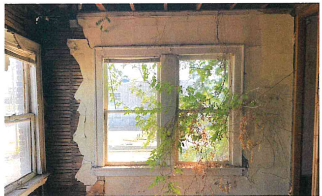
Daylight is coming through the wall in the top left corner of this room.
