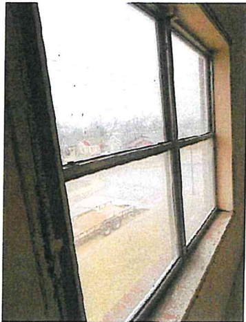
West Side Replacement Window- 3 (single pain window with aluminum track and spring balancers
