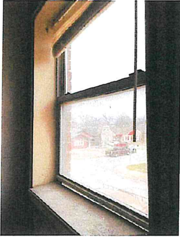
West Side Replacement Window- 2 (single pain window with aluminum track and spring balancers
