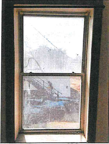
Back Replacement Window- 1 (single pain window with aluminum track and spring balancers)
