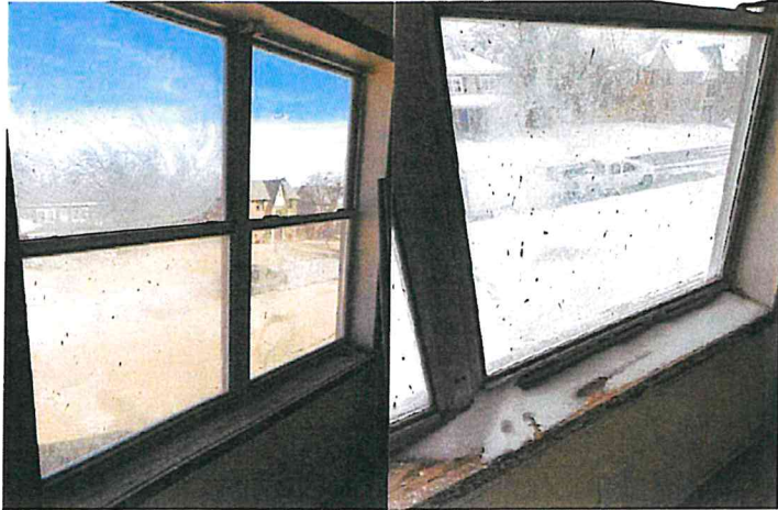
Front Replacement Window (single pain window with aluminum track and spring balancers)
