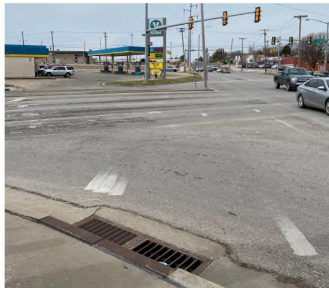
Photo 2: Worn Crosswalk Pavement Markings (South leg of NW 10 th & Virginia)
