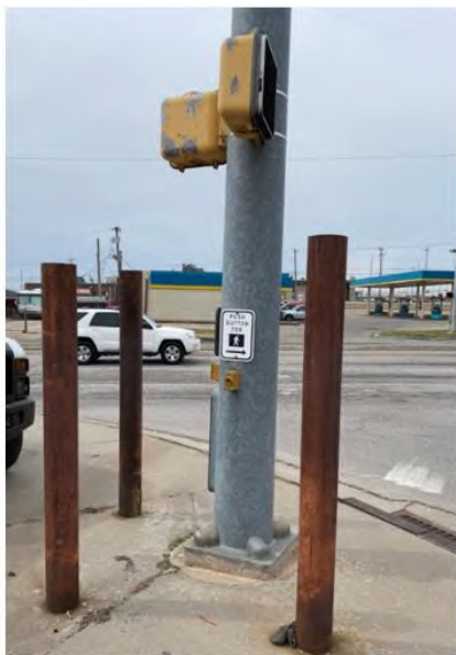
Photo 1: Inaccessible Pedestrian Pushbuttons (Southeast corner of NW 10 th & Virginia)
