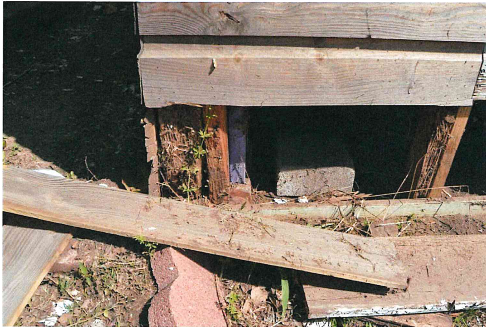
#5: Condition Assessment: January 2021 (Preservation and Design Studio) Close-up of termite damaged stud structure.
