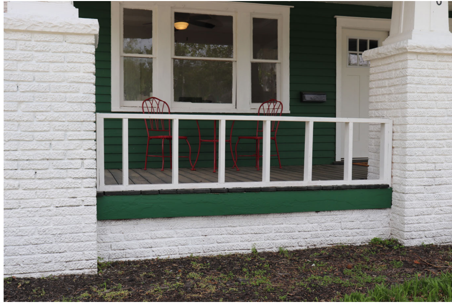
North (front) Porch Railing Replacement
