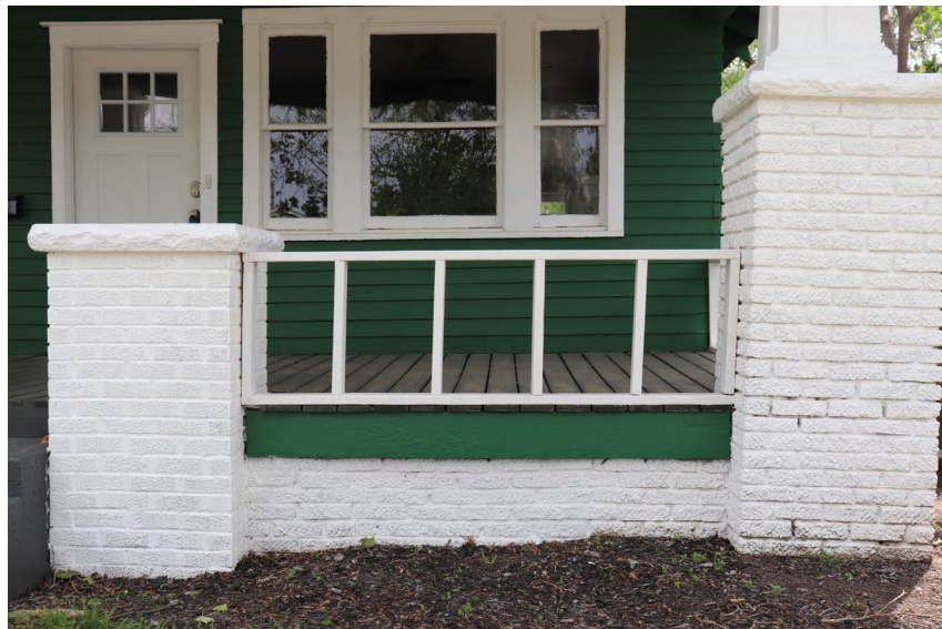
Pier Reconstruction and Railing Replacement
