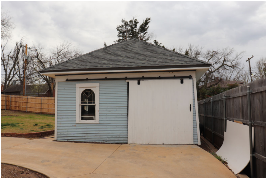
North Façade of Garage with Replacement Sash in Window Opening; Note West Wall
