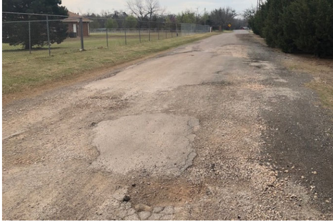
Photo taken 3.27.21. Damage to Hassett Road and attempted filling of potholes with gravel
