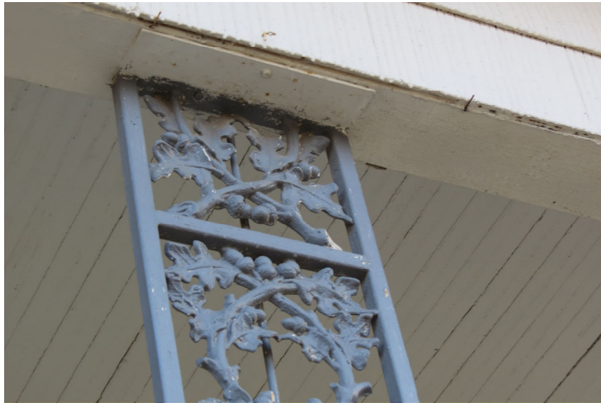
Plate Attachment of Column to Front Porch Beam; no obvious indication of previously existing column
