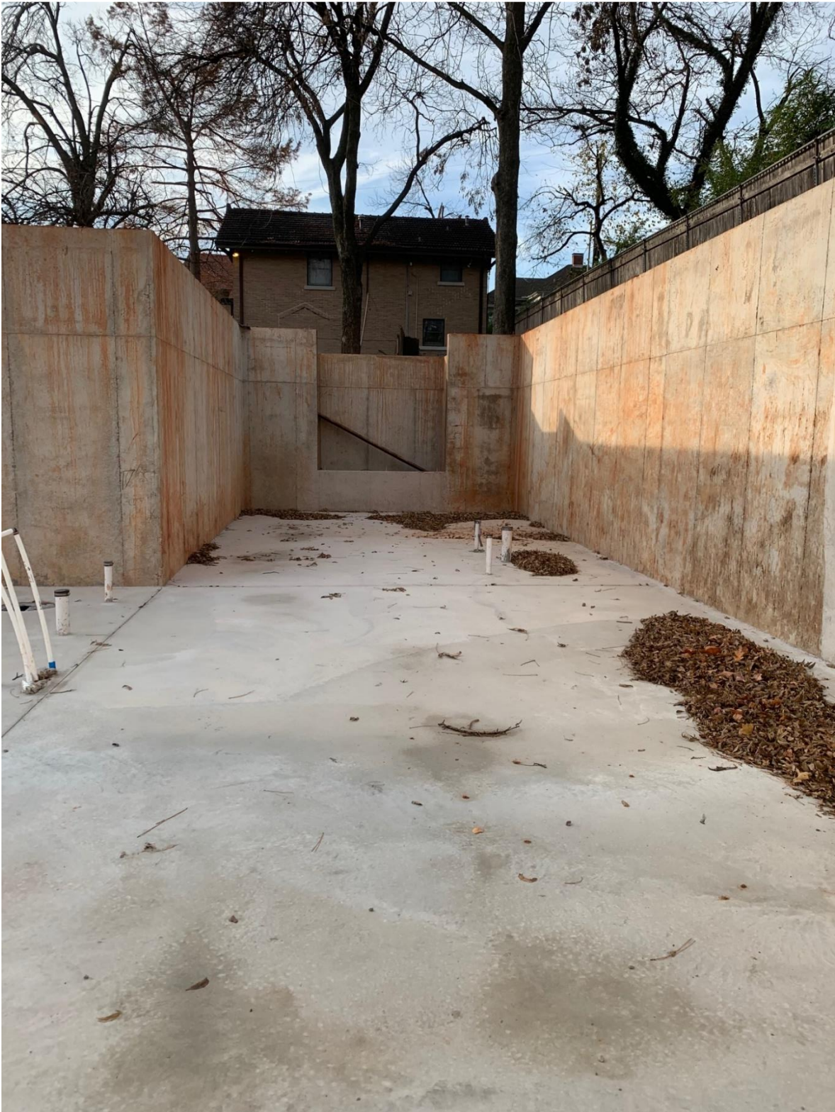
Window well on south wall (before framing)
