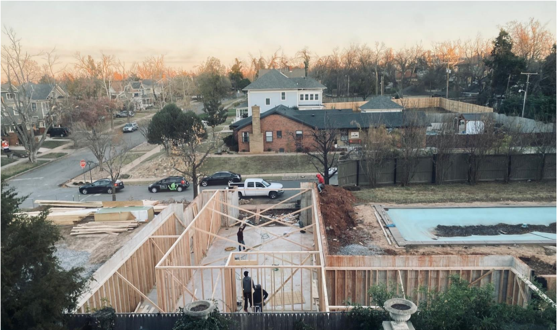
Overhead view of basement framing
