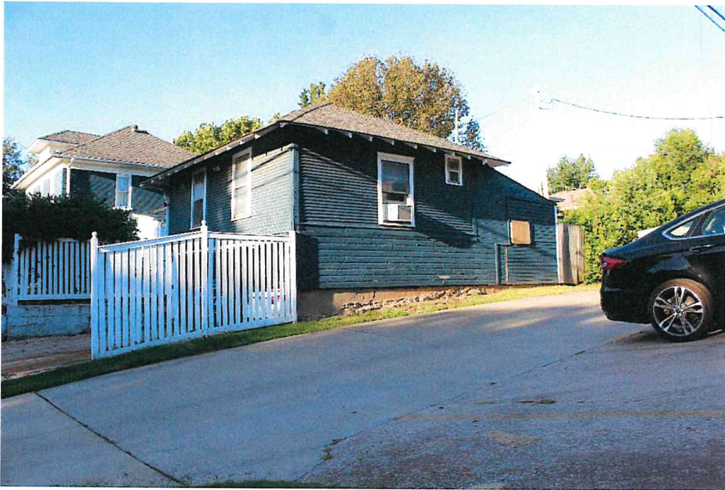
East facing façade (left) and north elevation. Two-story east section with hipped roof (left) and one-story, west section, addition with shed roof. (August 2020, PandDS)
