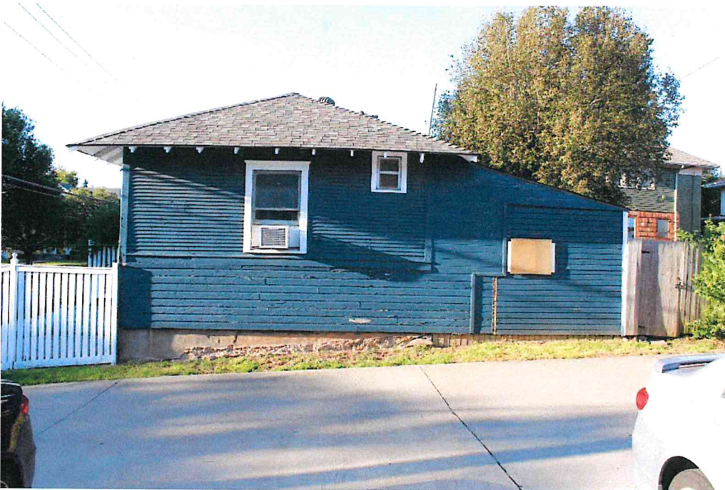
North elevation. Two-story east section with hipped roof (left) and one-story west section addition with shed roof. Wood lapped siding on the second floor of the east section has 3" exposure and drop siding along the rest of the elevation with 5" exposure. (August 2020, PandDS)
