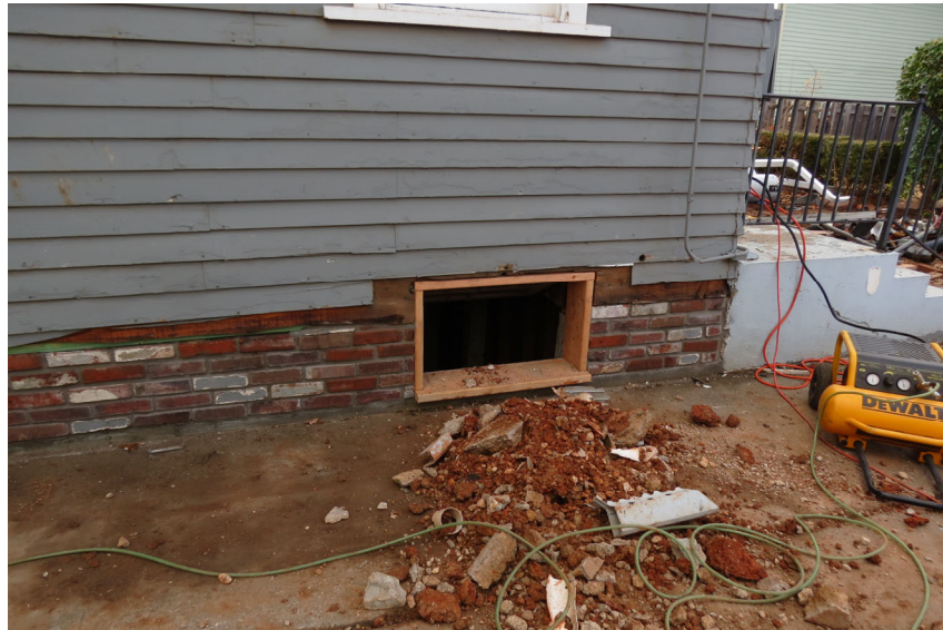
Basement Window Opening and Brick Stem Wall
