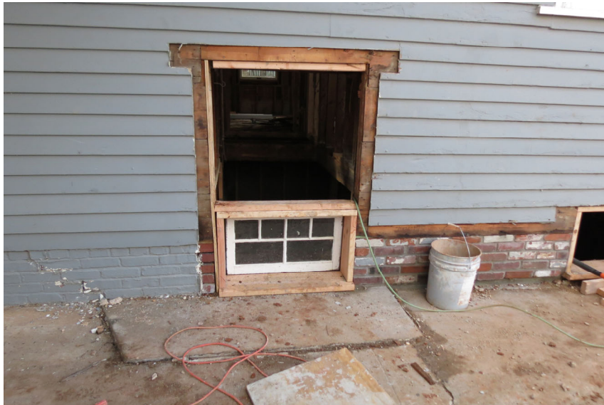
Basement Door Opening with Window Installation Depicted
