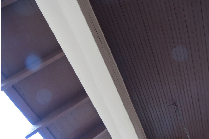
Porch Beam Above East Pier Offers No Evidence of Previously Existing Column
