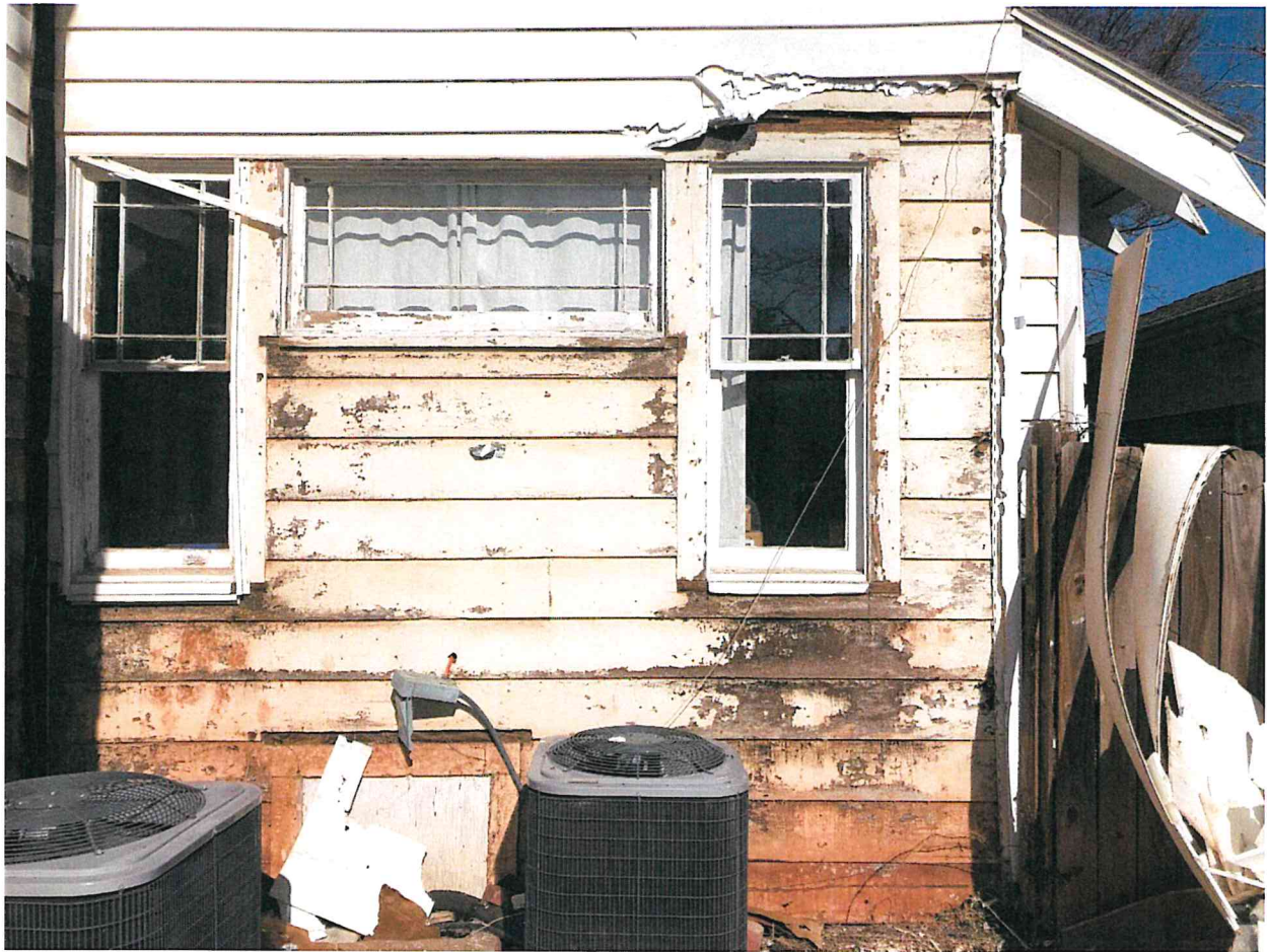
South/East Elevation – original wood revealed before removal of 50% of one side as per guidelines. All missing trim was removed and window sill ends cut in the vinyl installation and will be restored with appropriately sized and sourced material.
