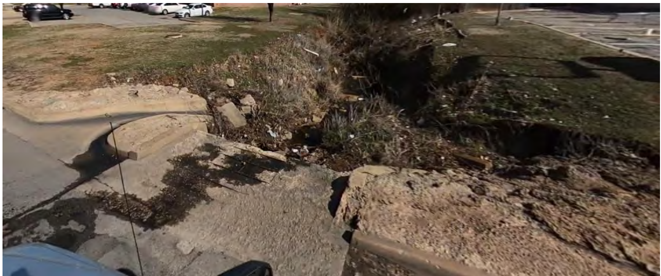
Image 6: Drainage Structure on Lyrewood Lane showing signs of distress. Location near Knight Lake Drive and Lyrewood Lane.
