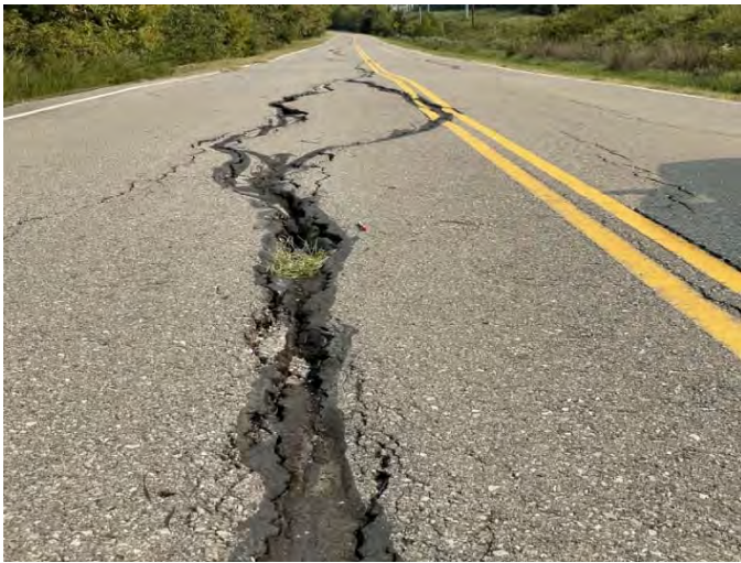
WM-0343 – Widest Longitudinal Cracking
