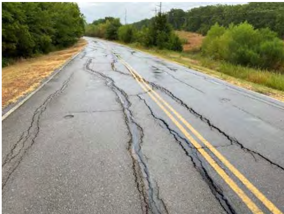
Photo 3 – Pavement condition near approximate location of boring B-7E
