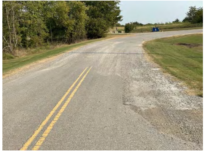
WM-0342 Pavement Deterioration
