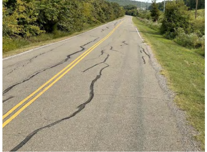
WM-0343 – Longitudinal Cracking
