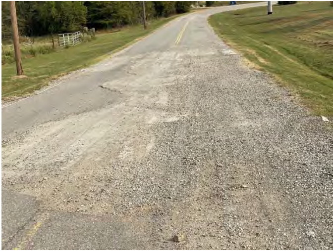
WM-0342 Pavement Deterioration
