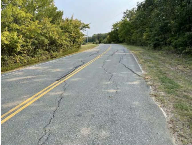
WM-0343 – Longitudinal Cracking
