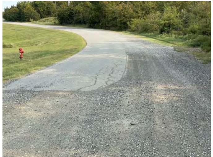
WM-0342 Pavement Deterioration
