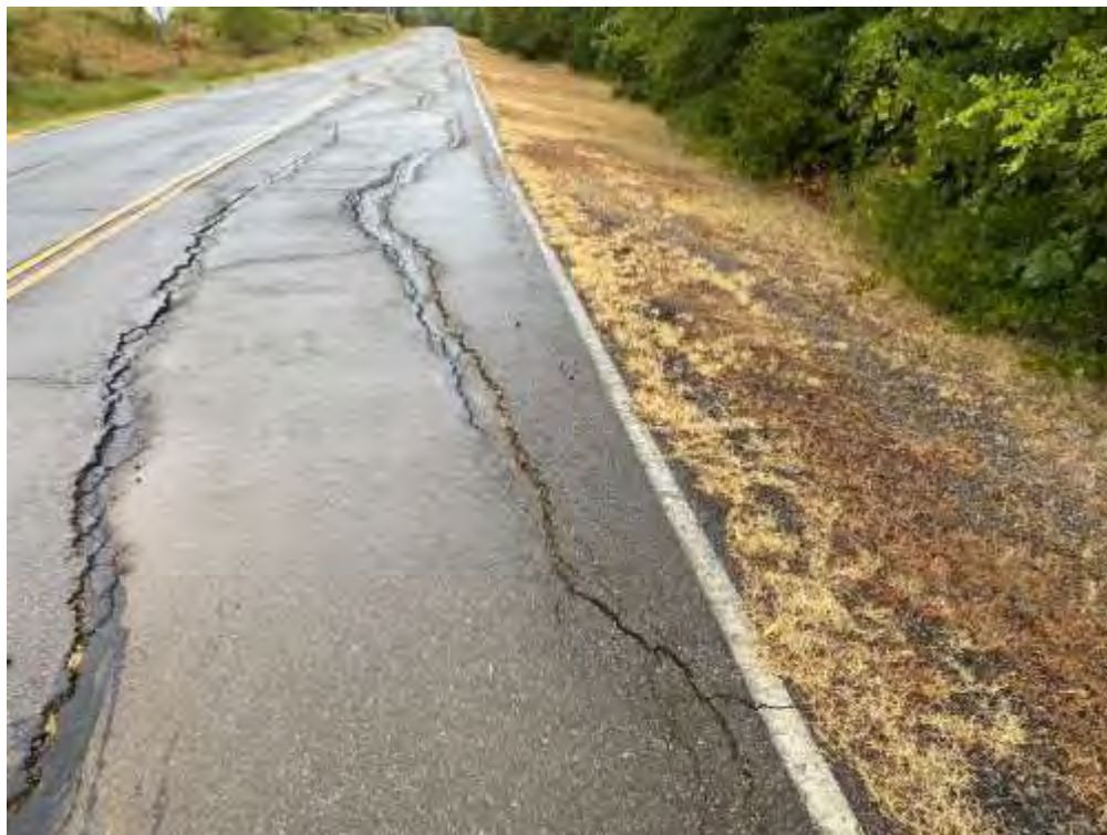
Photo 5 – Pavement condition near approximate location of boring B-7D
