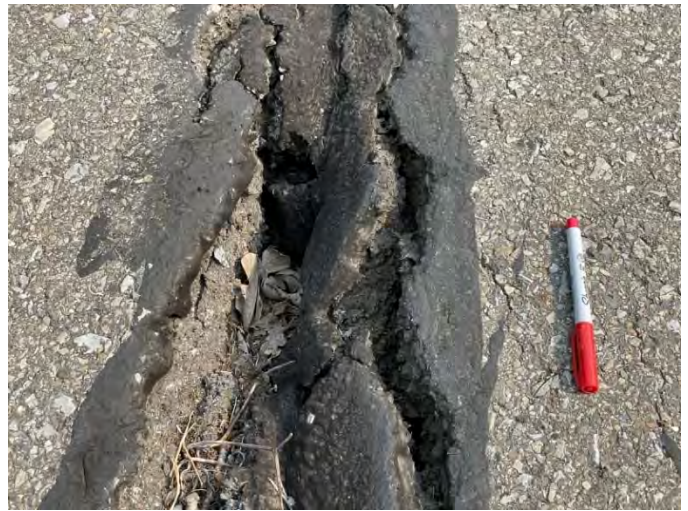
WM-0343 – Widest Longitudinal Cracking
