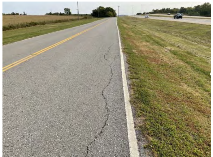
WM-0342 – Pavement w/ Longitudinal Cracking
