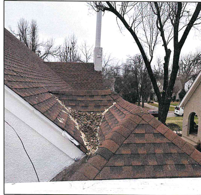
Existing roofline has a drainage issue to its current configuration. Project proposed to reframe this roof as a gable to match the south corner, terminating into the new proposed dormer. Allowing the proposed extension to shed water properly.
