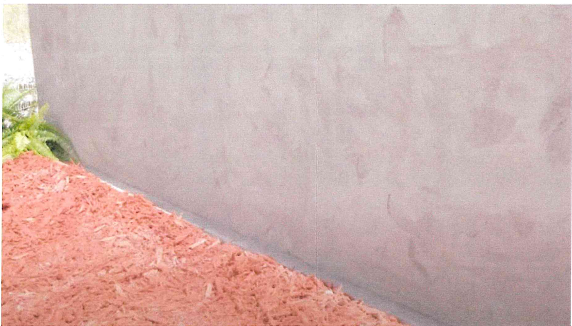
Parged Concrete at Existing and New Retaining Walls (Painted to Match EN-V-011 Charcoal or Similar)
