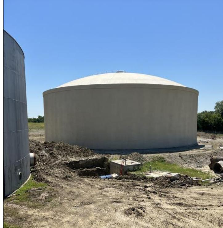
In the last 2 years we have replaced two of the three balancing tanks on the south end. There is one additional tank that will be constructed in a later phase of the new pipeline construction.
