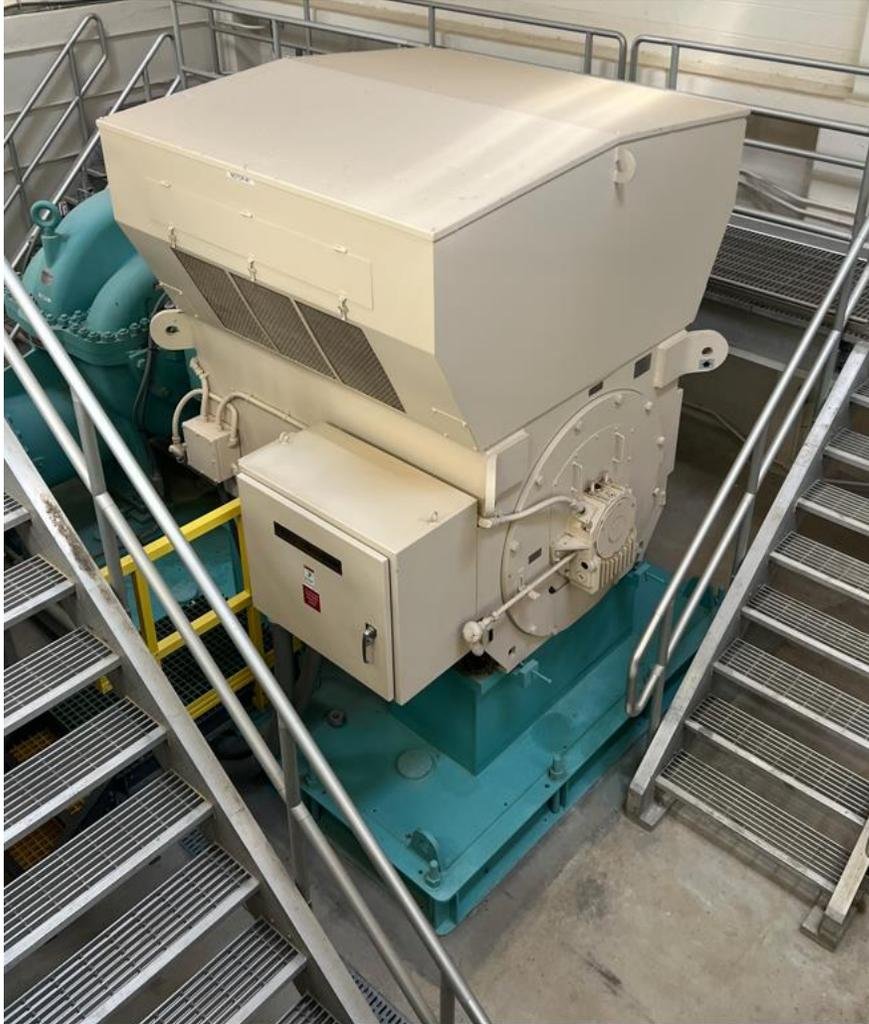
Currently we are running extensive PDMA quarterly testing on our electric motors and all are in good condition. Our electric motors are still performing within factor specifications.
