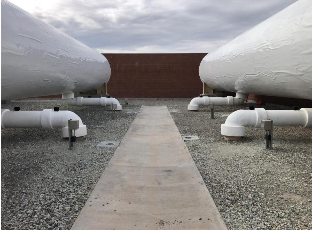
Our surge system has been online roughly 3 years and has been deployed during some of our severe weather power outages. This system prevents major line breaks and is working as designed. With this added layer of protection, we are safeguarding against line breaks, ensuring consistency in pumping operations, and preventing costly line repairs.
