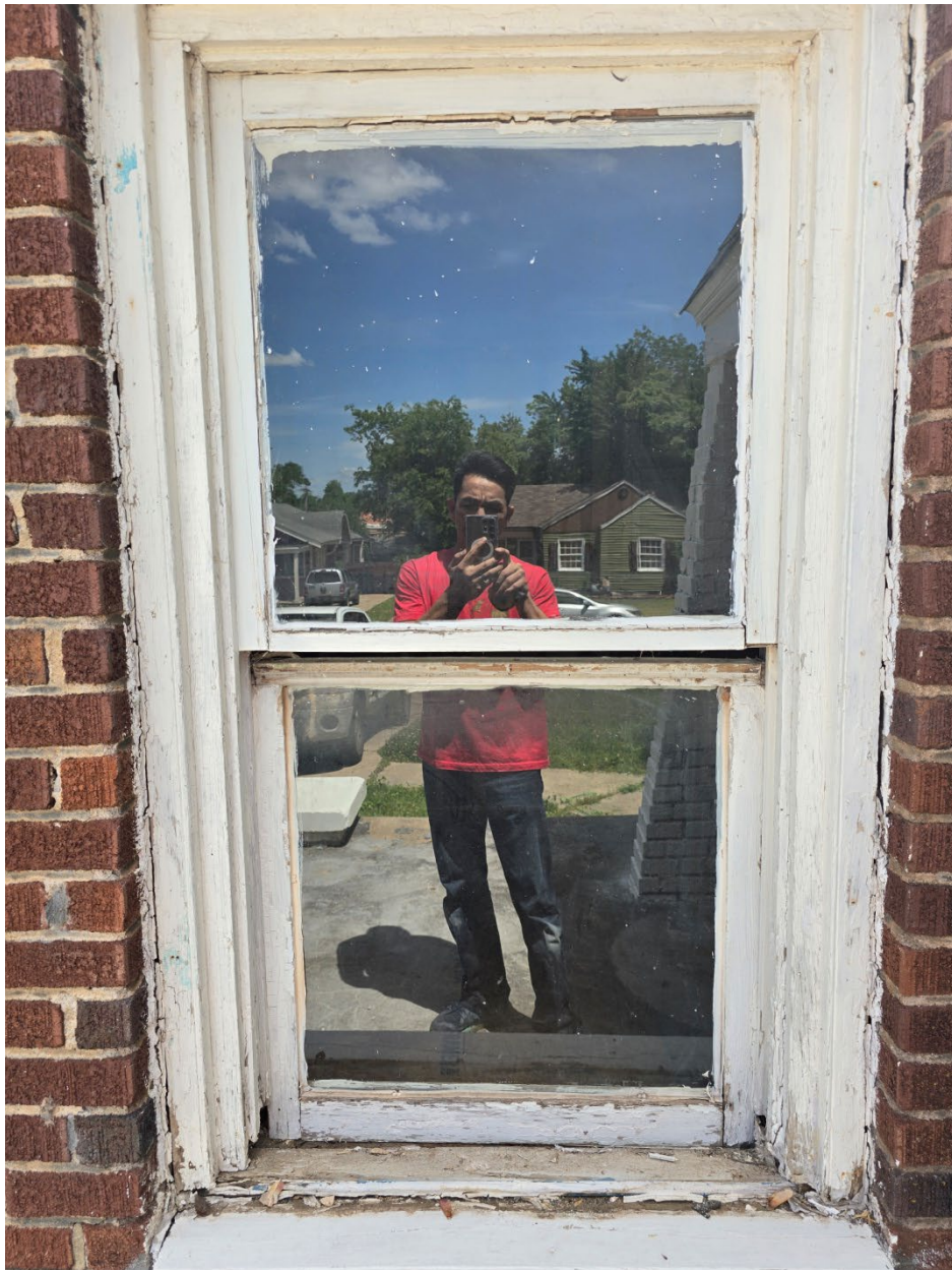
Window # 5 – 28 x 54 – Left front in porch area Too damaged to repair, propose to replace
