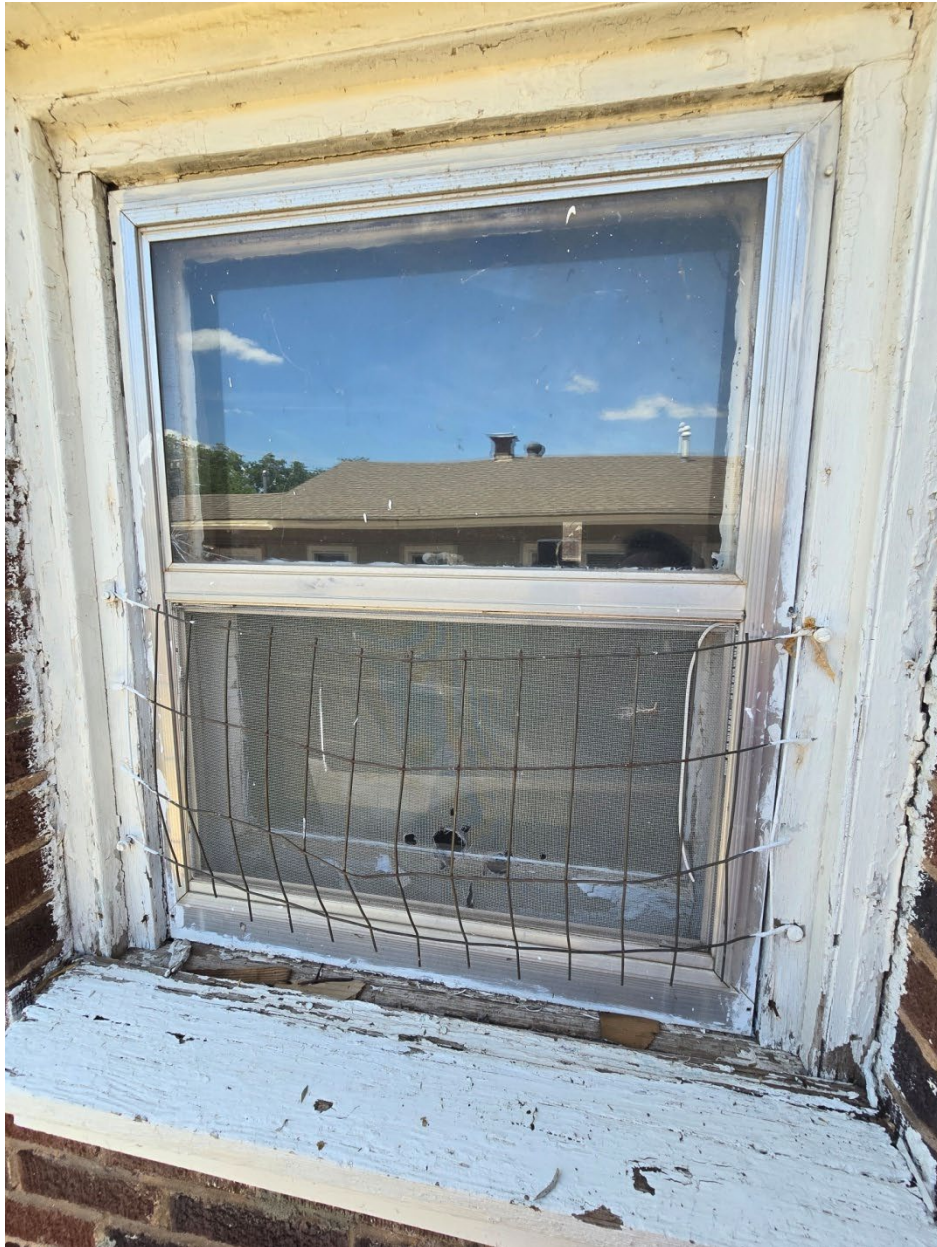
Window # 8 East side of house bathroom – Too damaged to repair, proposed to replace
