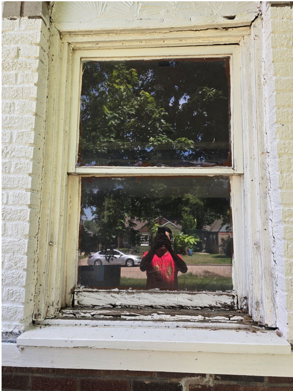
Window # 2 – 36 x 54 – Front Middle – Too damage to repair, propose to replace
