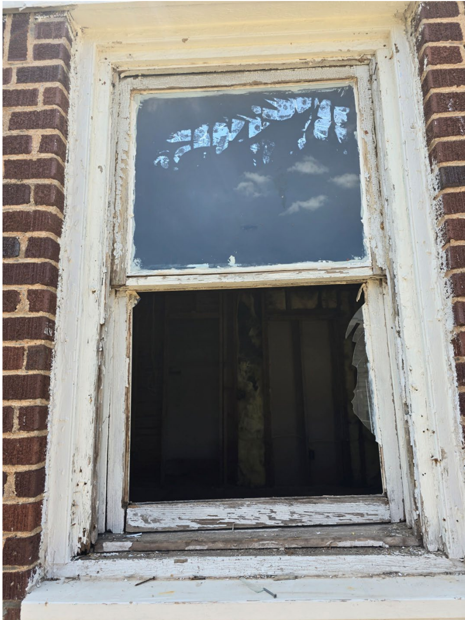
Window # 6 – 32 x 54 – Too damaged to repair, propose to replace
