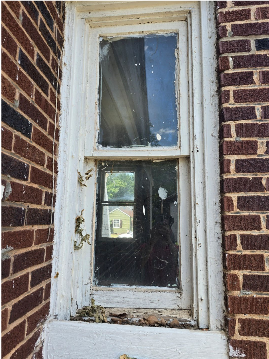
Window # 7 22 x 54 – Too damaged to repair, propose to replace
