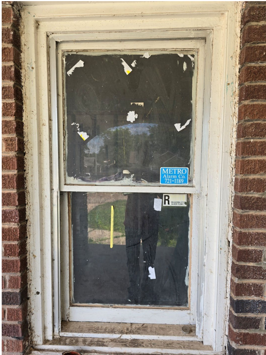
Window #4 – 28 x 54 - Front left side in porch area – Too Damage to repair, propose to replace
