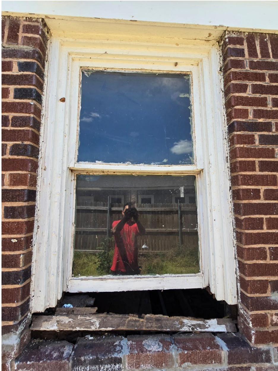
Window # 9 Southeast bedroom – Too damaged to repair, propose to replace
