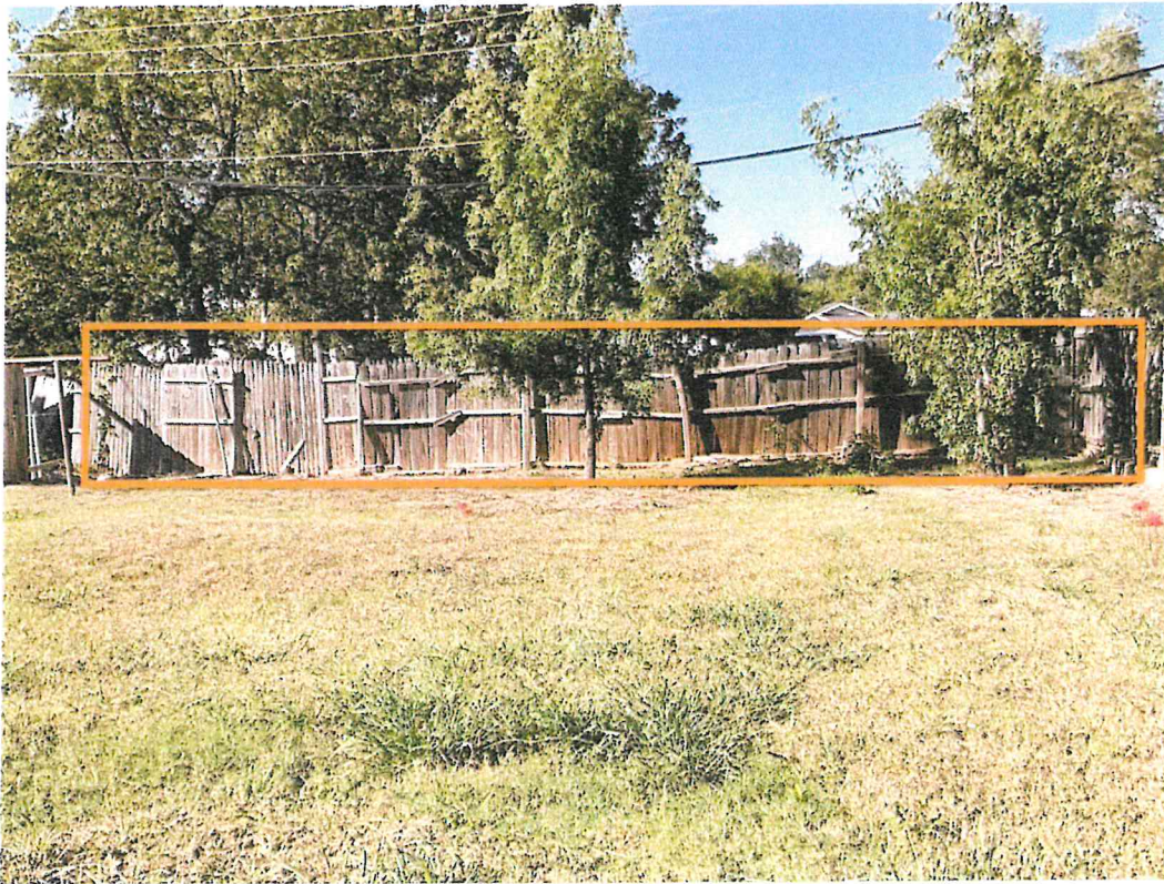
Figure 2: Dilapidated rear (west to east) portion of fence to be replaced with new fence
