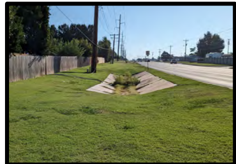
Figure 25: S.W. 134 th St. Paved Ditch
