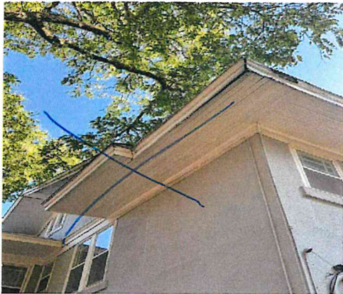
Existing, rotted eaves. Picture shows existing crown moulding that is incompatible with the installation of new gutters.
