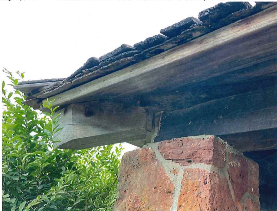
Photograph #4 – Deterioration of cedar shakes and heavy timber
