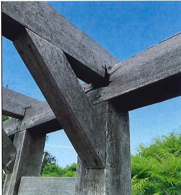
Photographs #9 & 10 – Heavy Timber damaged and out of plane
