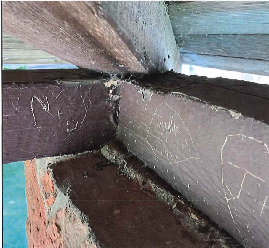
Photograph #3 - Interior corner detail showing deteriorated heavy timber framing.
