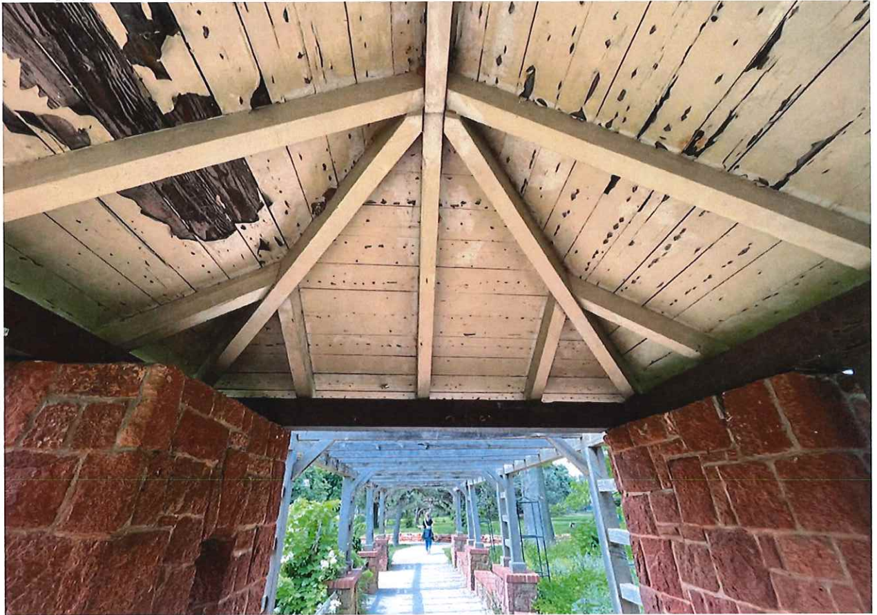
Photographs #11 – Water damaged roof deck
