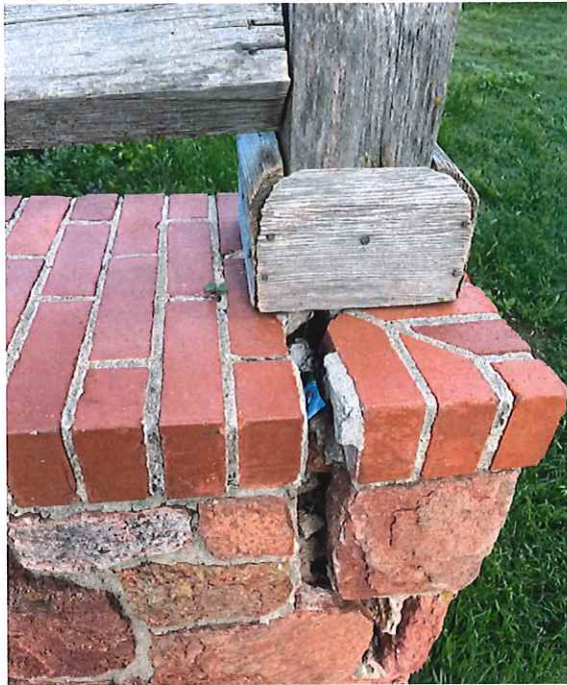
Photographs #7 & 8 – Water damaged masonry
