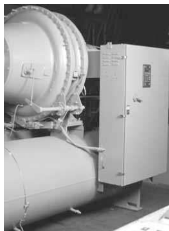
Figure 20. Starter mounting bracket
