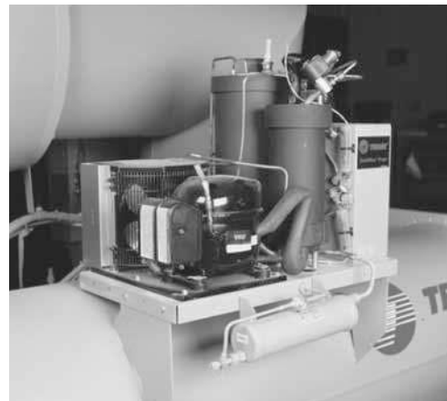
Figure 6. Purge unit detail
