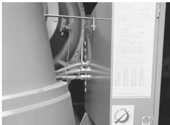
Figure 18. Control panel mounting bracket
