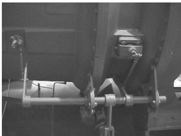
Figure 12. Vane actuator operator mechanism
