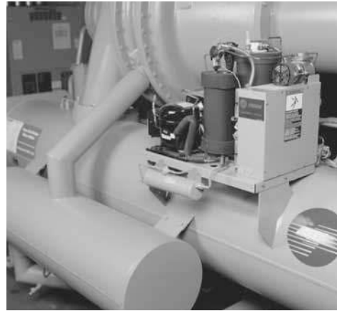
Figure 5. Example purge unit
