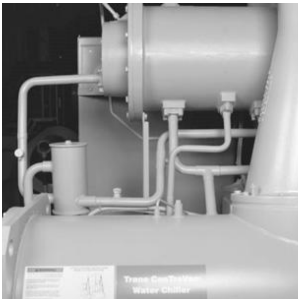
Figure 14. Lubrication system motor cooling lines
