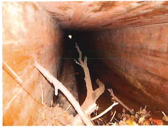
Figure 21 - Anchored 10" SS in box
