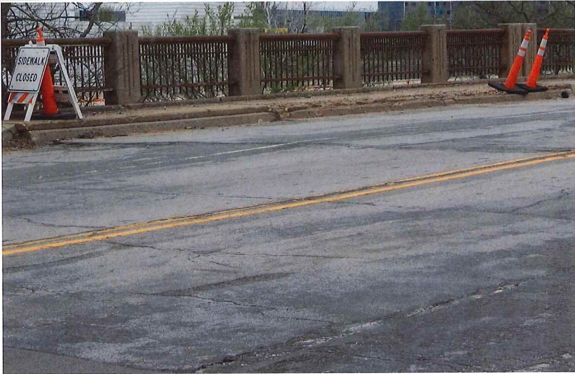
Figure 3 - Typical Condition of Pavement East of Bridge
