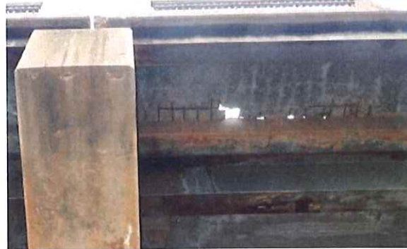
Figure 8- Opening in Sidewalk and Exposed Rebar
