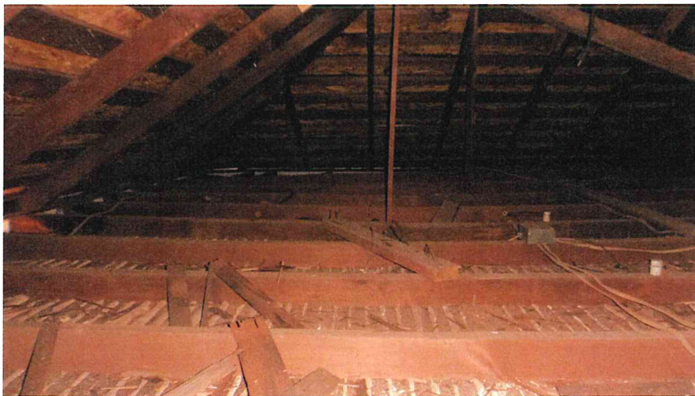
Signs of previous fire in attic. No insulation in attic.
