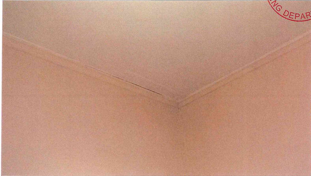
Water damaged ceiling
