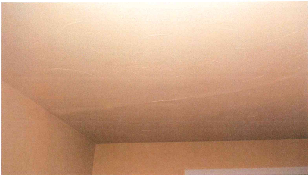
Ceiling cracking.
