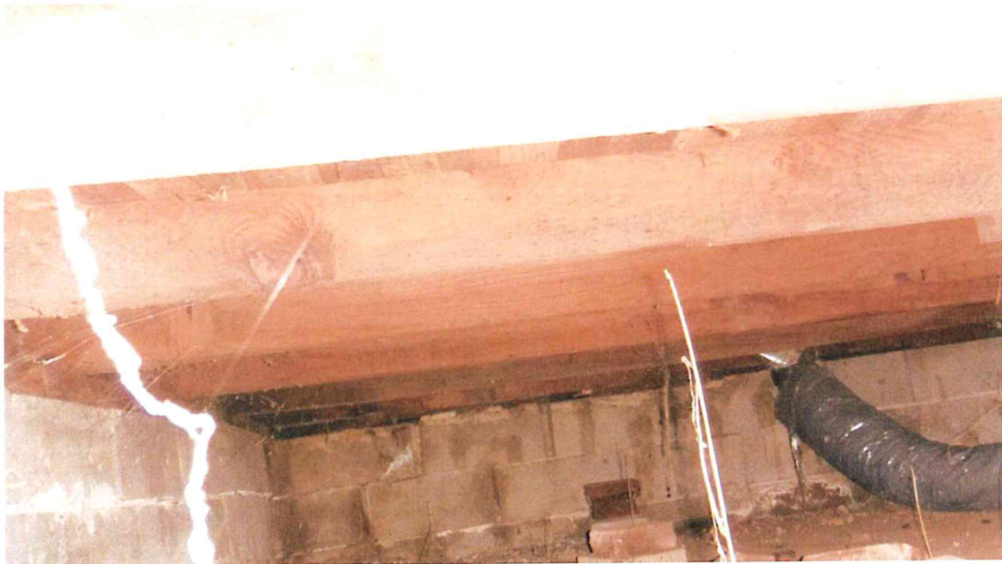
West foundation wall from crawlspace. Block knocked out of alignment or broken bond.
