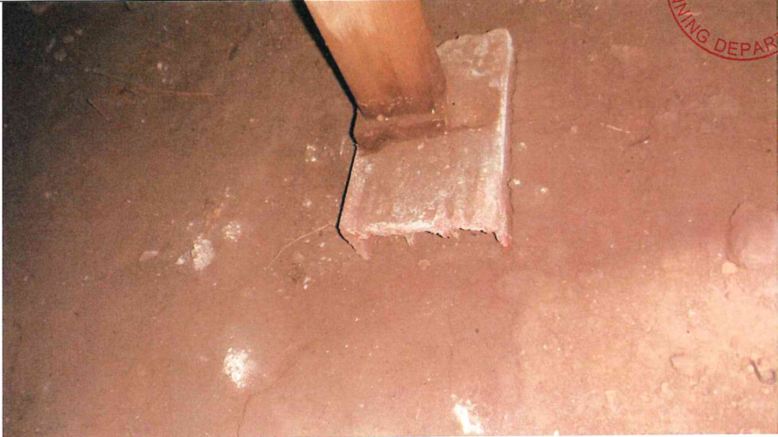
Clay brick support for post and beam. Partially sunken.
