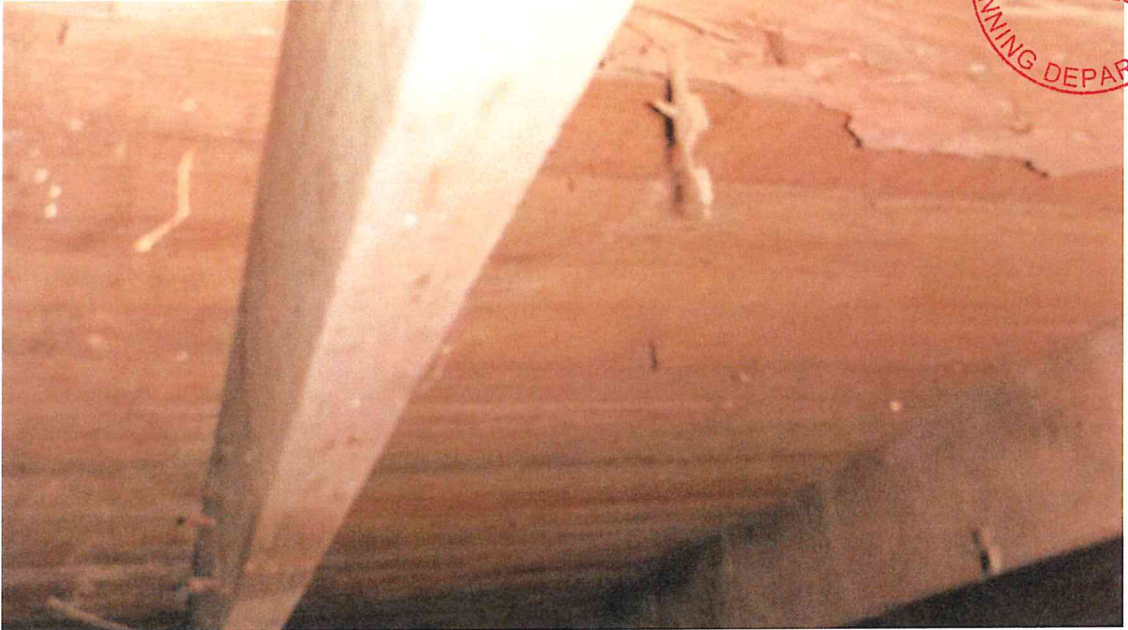
Split sub-floorboards and termite damage evident.
