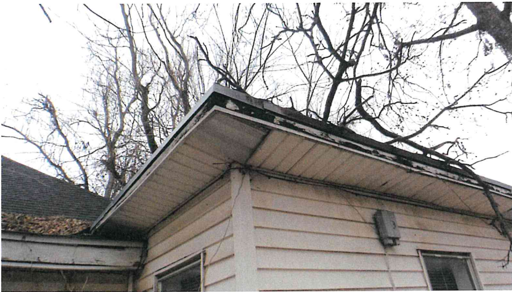
Roof damage from falling tree branches.
