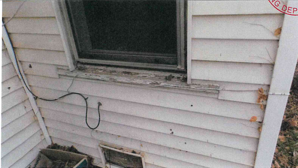
Rotting window sills.
