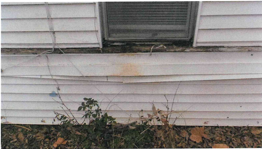
Rotting wood at windowsills all around the house.
