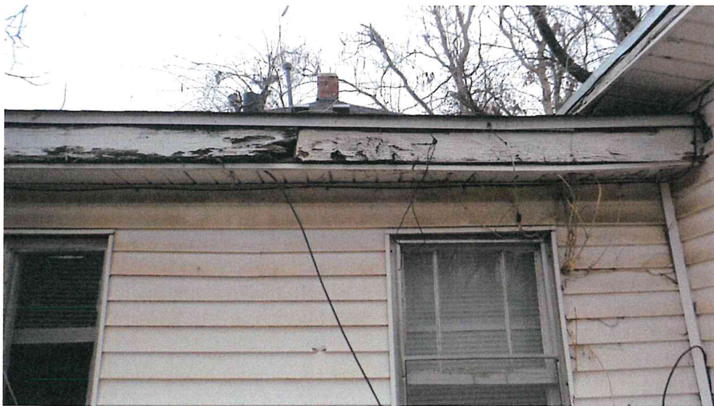
Rotting fascia. Plants growing out of siding.
