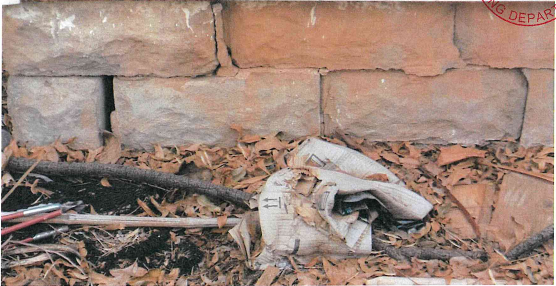
West foundation wall blocks out of alignment and movement evident.
