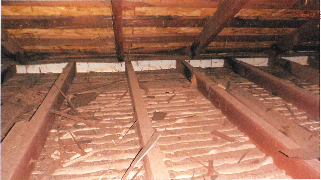
Construction debris left from previous sheathing replacement.
