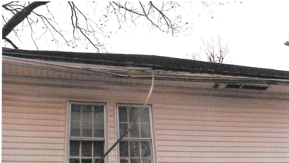
Roof damage at front of building from tree branches.
