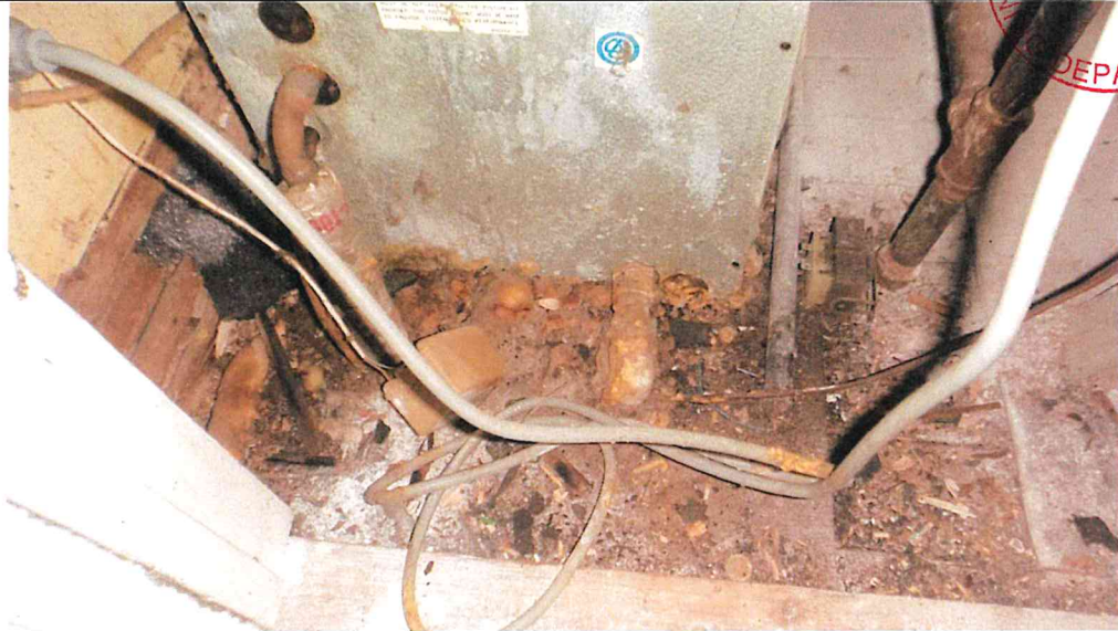
Evaporator unit for AC is badly corroded.
