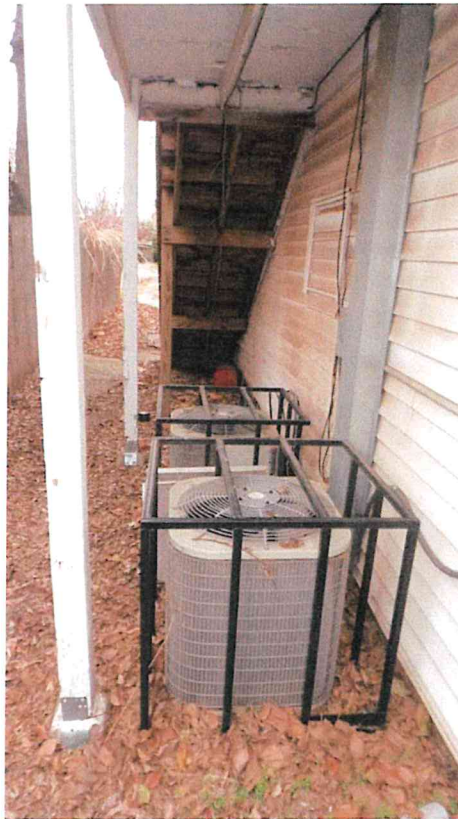
AC Compressor units under stairs in cages.
