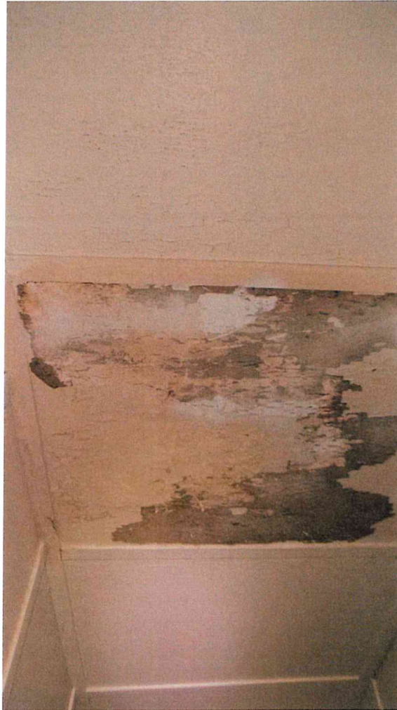
Ceiling panel in closet has water damage.
