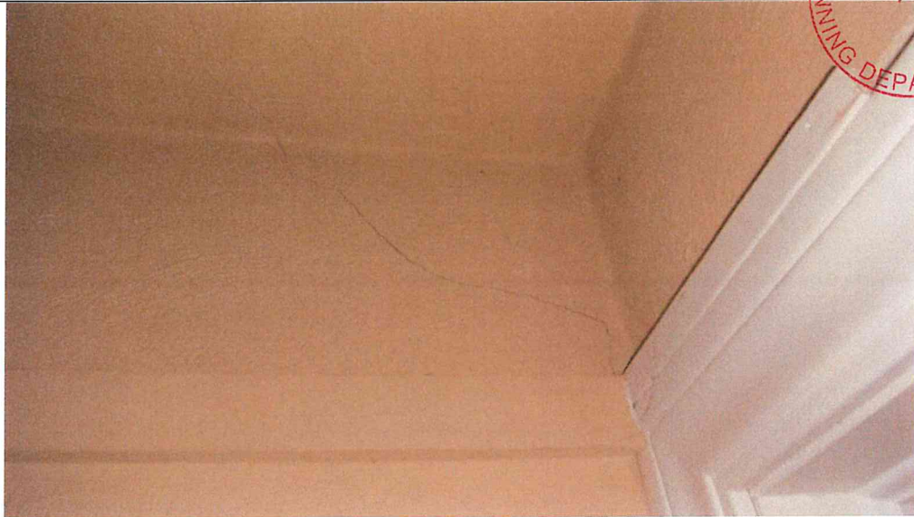
Wall cracking at corners
