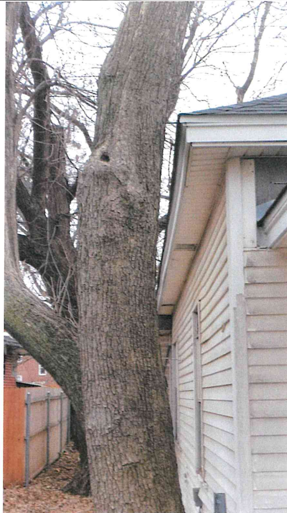
Tree at NE corner of house growing out of foundation base.
