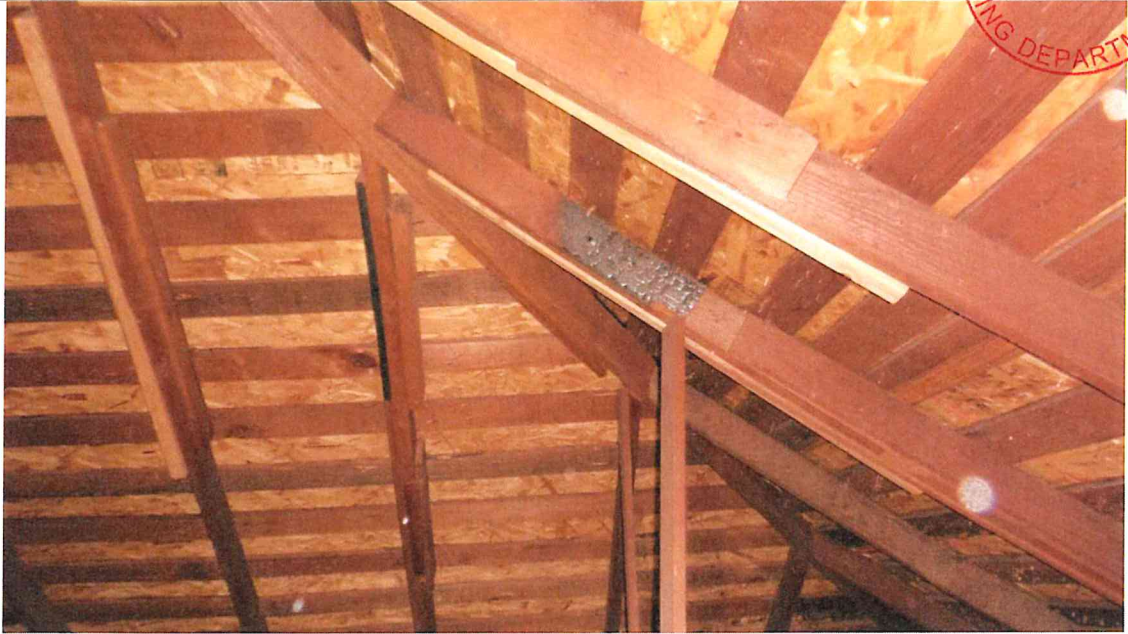
Previous repairs to rafters and recent addition of wind bracing.
