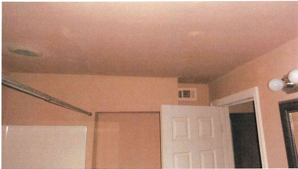
The ceiling shows warpage from water leakage in bathroom.
