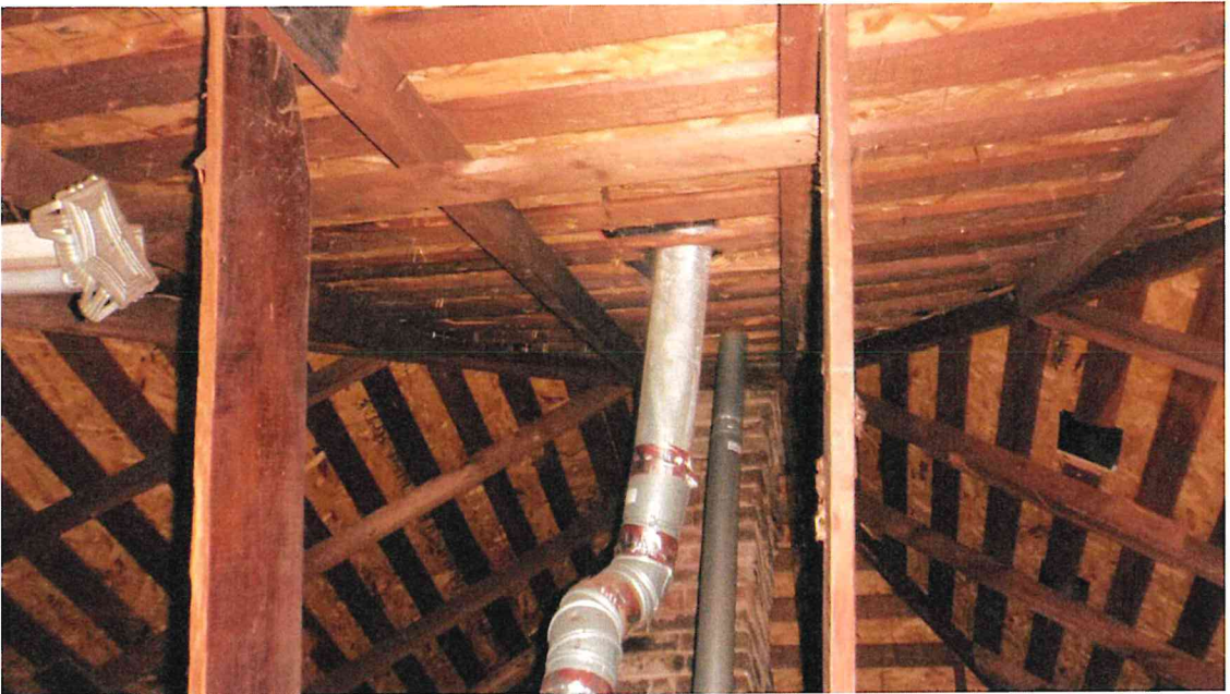
Charred framing in attic. Significant sagging of roof.
