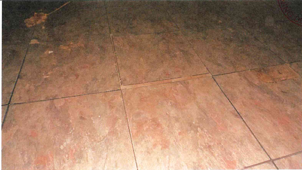
Tiles unbonded and loose.
