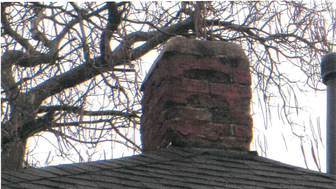
Decomposing brick and mortar of chimney at center of house.
