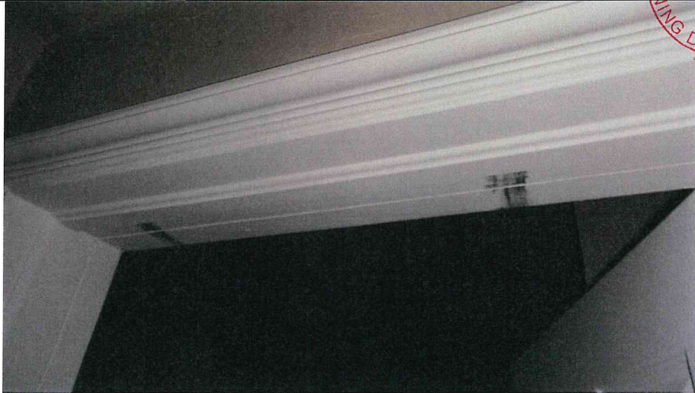
Door rub marks from building uneven settlement.
