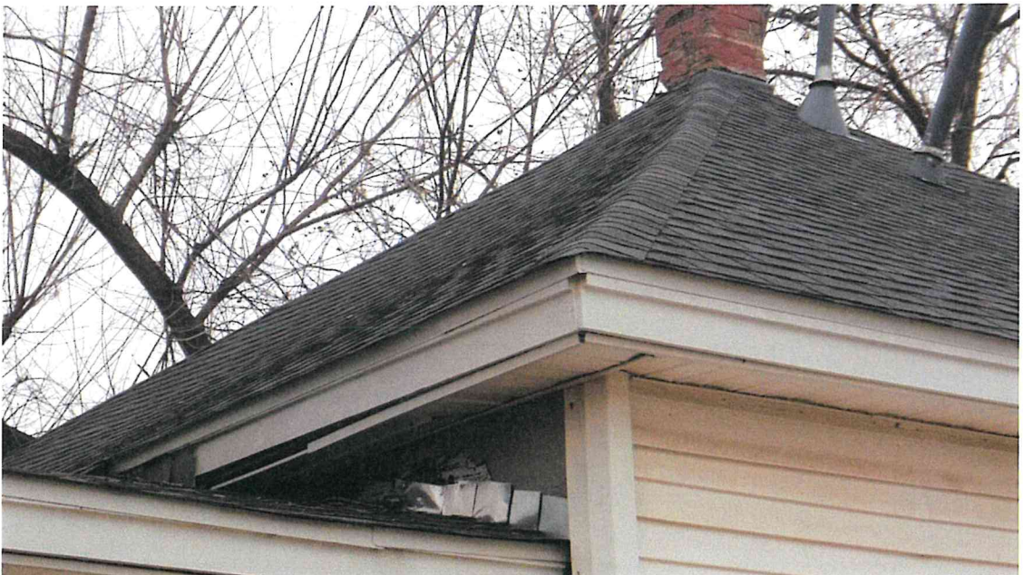
Roof sagging evident.
