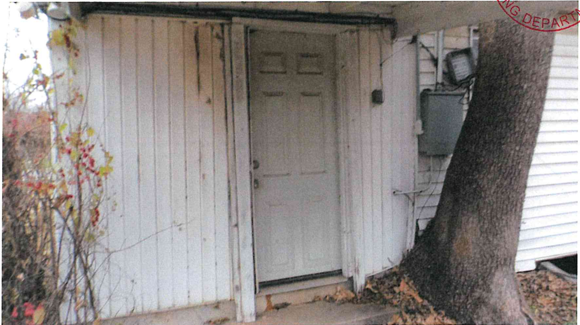
Tree growing out of base of foundation and causing floors to heave.
