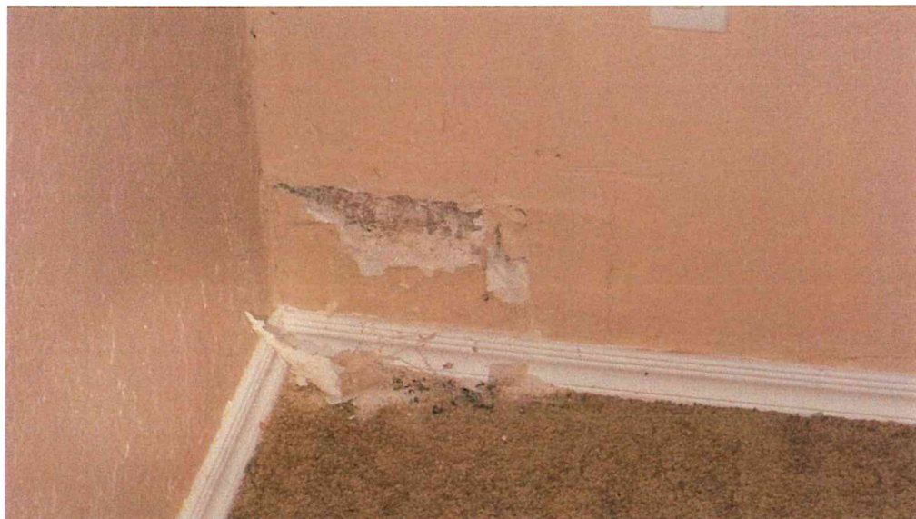
Water damage from floor up wall in front room.
