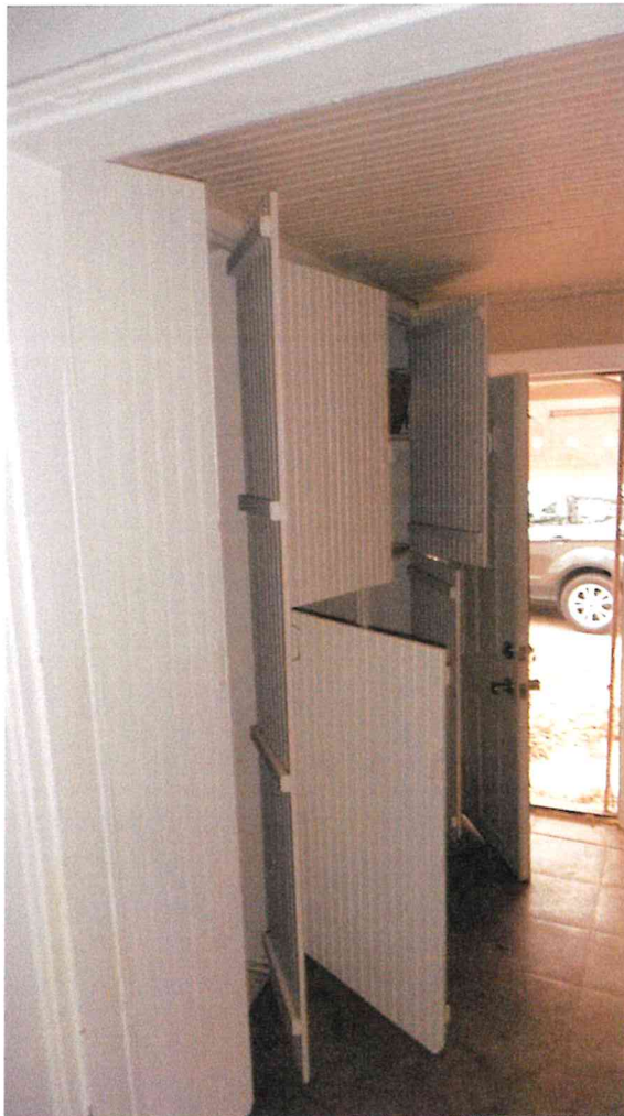
Doors in utility room cabinets swing open due to non-level floor.
