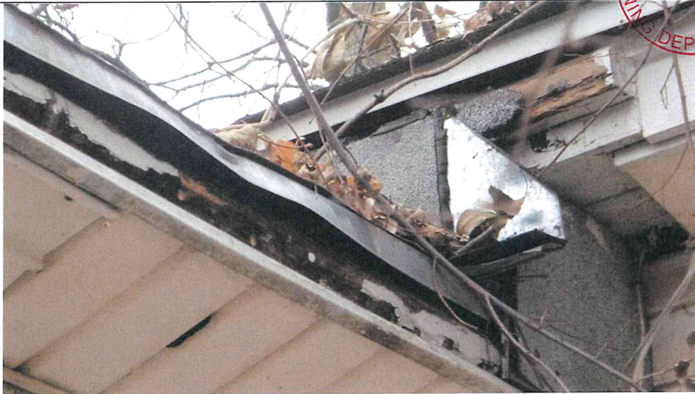
Damaged flashing and rotting wood at roof edges.
