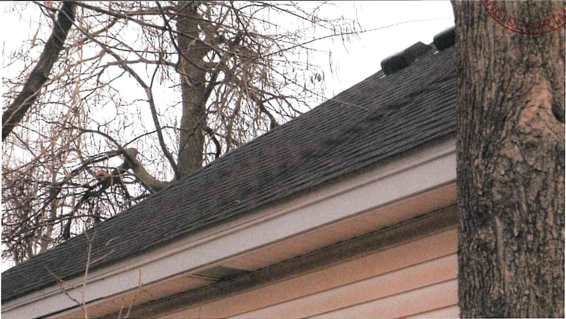
Roof sagging on all four faces of hip roof.
