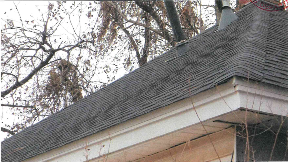
Roof sagging evident.
