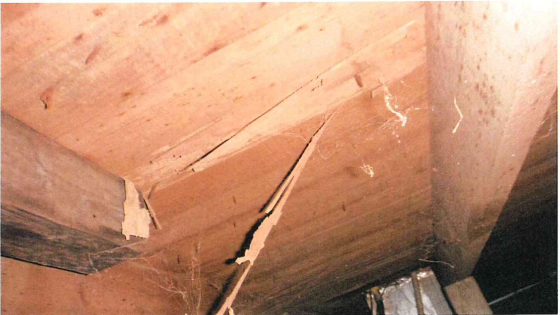
Split sub-floorboards and termite damage.
