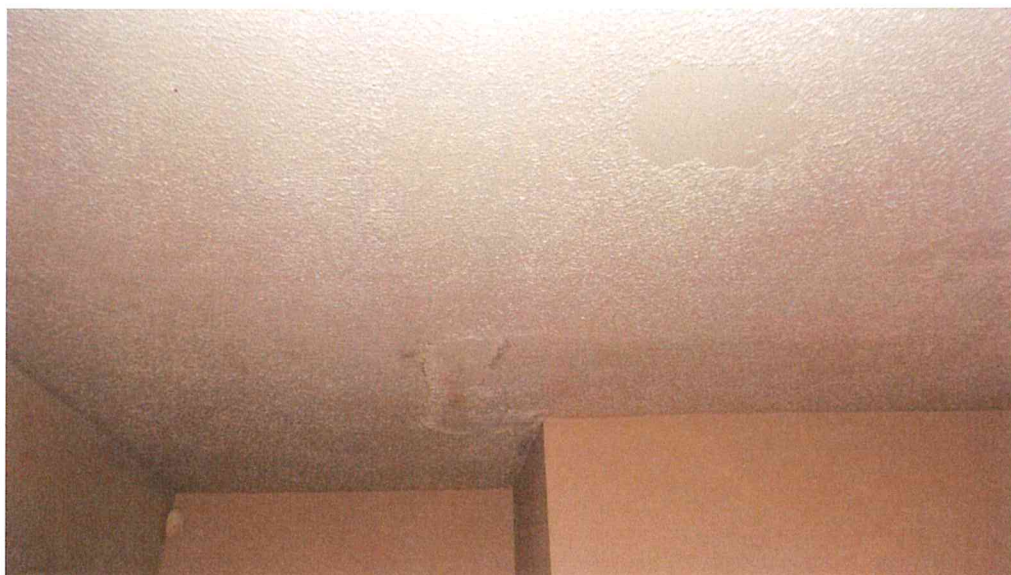
Water damaged ceilings.
