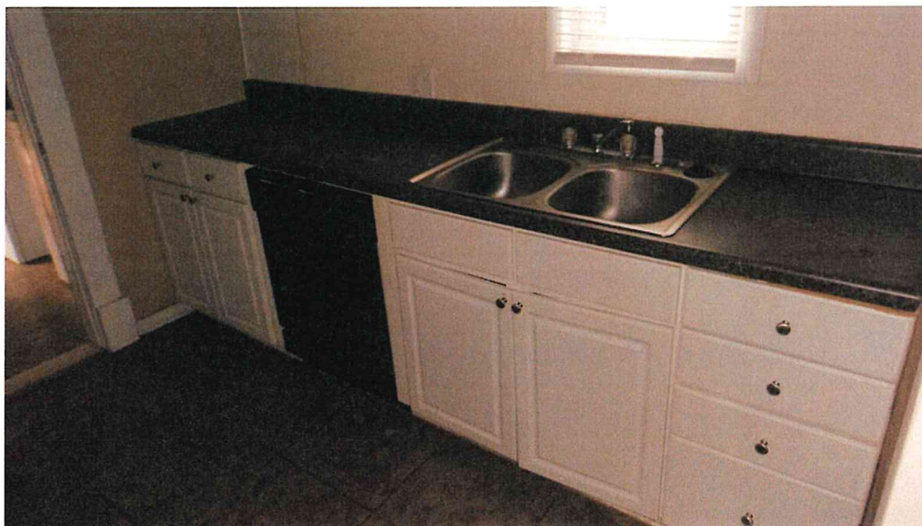
Newer cabinets installed over sagging floor.
