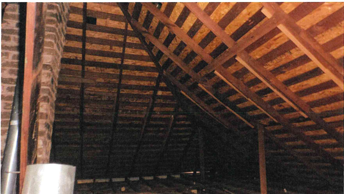
Sway of roof deck evident in attic.
