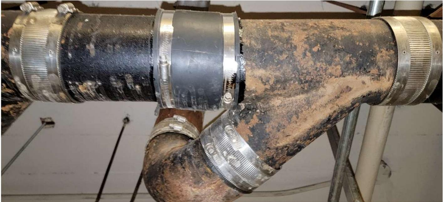
Figure 2. Possible Leak Allowing Sewer Gas to Enter Building
