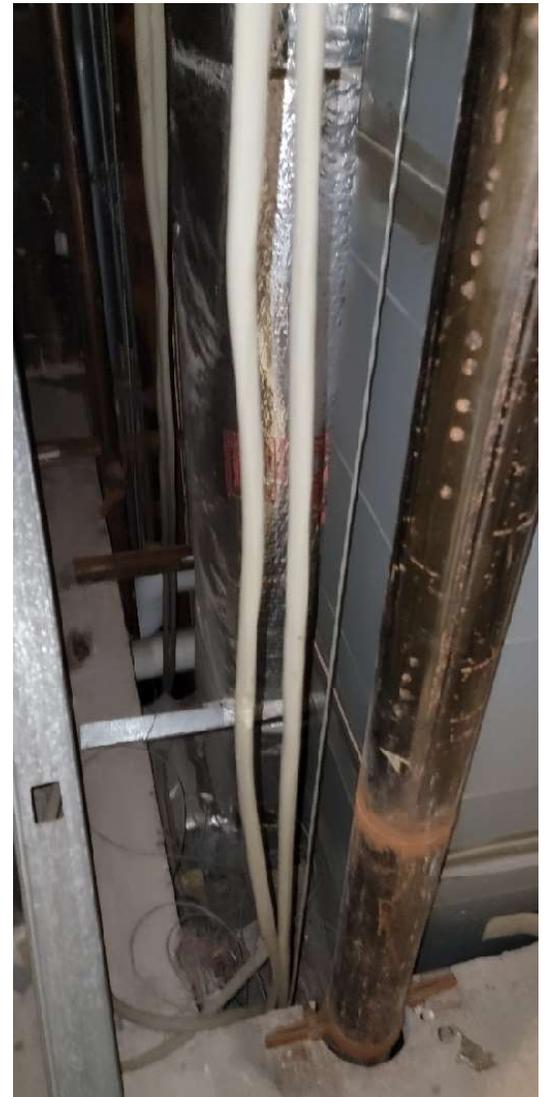
Figure 1. Typical Light Rust on Cast Iron Pipe
