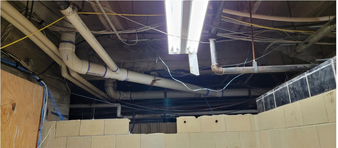
Figure 4. Sanitary Replacement Showing Use of PVC Pipe
