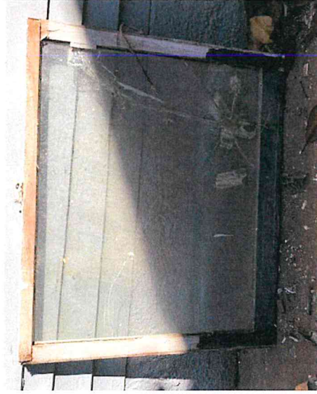
Documented bottom sashes that are not linked to an upper sash.
