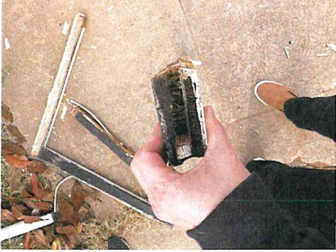
Additional photos of condition of bottom sashes. Significant rot and decay.
