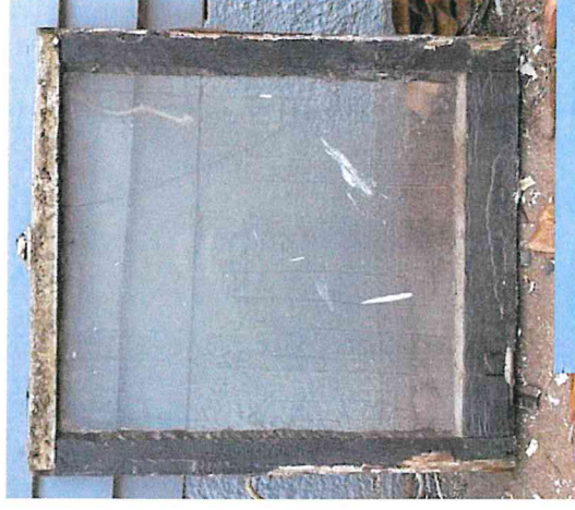
Documented bottom sashes that are not linked to an upper sash.
