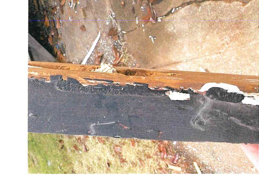
Additional photos of condition of bottom sashes. Significant rot and decay.
