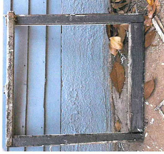
Documented bottom sashes that are not linked to an upper sash.
