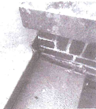
Porch extension is separating and pulling away from the backs of the house.
