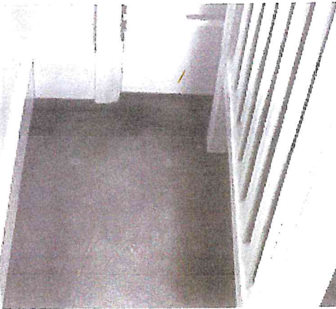
Stairs are deteriorating and create a blockade for water to sit and drain back towards foundation. This we believe has been causing the sidewalk to sink, as well as why we felt the porch extension is not original to the house.
