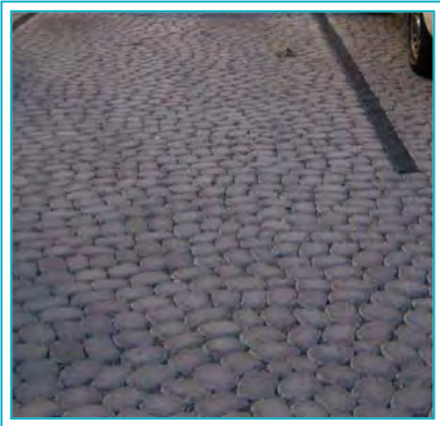
Parking lot with pervious pavers
